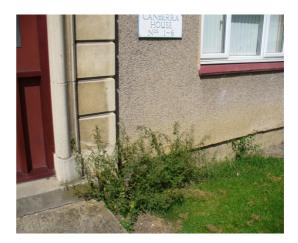
As well as weeds that are still alive there is evidence of weeds that appear to have been sprayed but have not been removed or not sprayed for a long period. Weeds in this category will appear to have been there for some time and there is little evidence that annual or routine maintenance has taken place.
